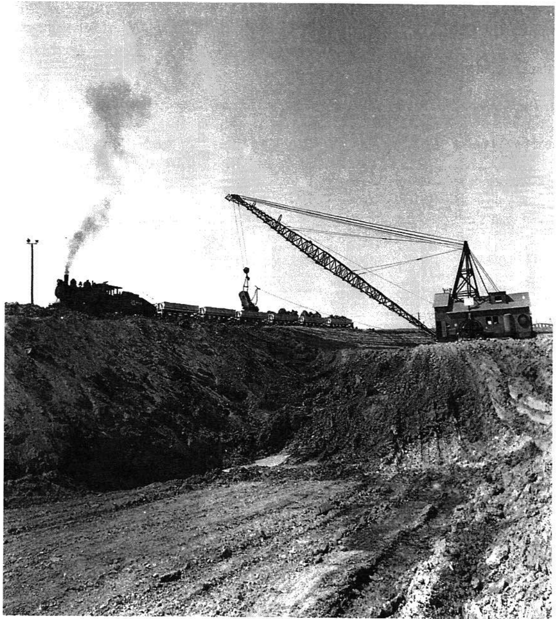
The drag-line crane shown here is the same type crane used in the rip-rapping project in Hog Jaw Valley. In this photograph it is excavating a large ditch.
